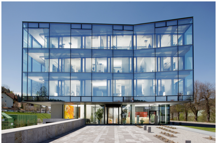
Testo-Headquarters in Lenzkirch, Foto: testo AG
